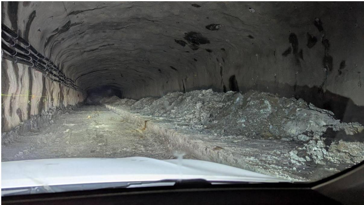
Picture 2: One chamber in the deep repository which is already filled with waste from the refinement process, but which has not been sealed yet. The mixed waste have a solid form and looks like a pile of gravel.
