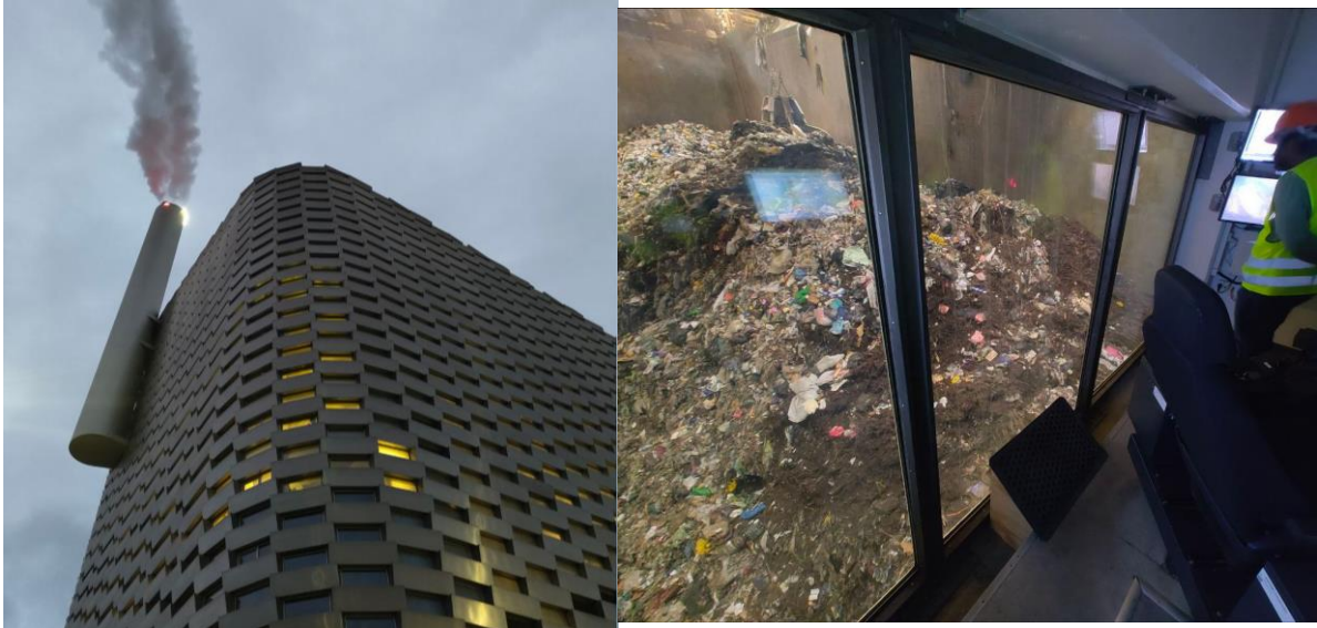
Figure 2: Left – Outside view of Amager Bakke from the parking lot. Right – Inside view of the control room for waste management
